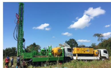
Water well drilling
